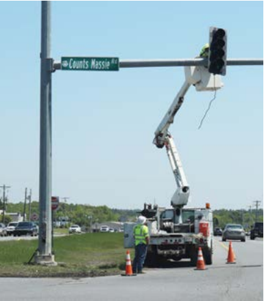
Updating a traffic signal to the current standard on Maumelle Boulevard. Photo courtesy of the city of Maumelle.
