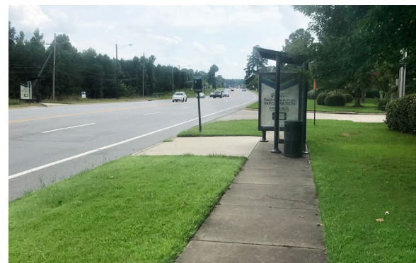
When Hwy 5 was widened in Little Rock, regional cross sections called for the inclusion of sidewalks and bike lanes. Rock Region METRO also added a bus shelter at this location.
