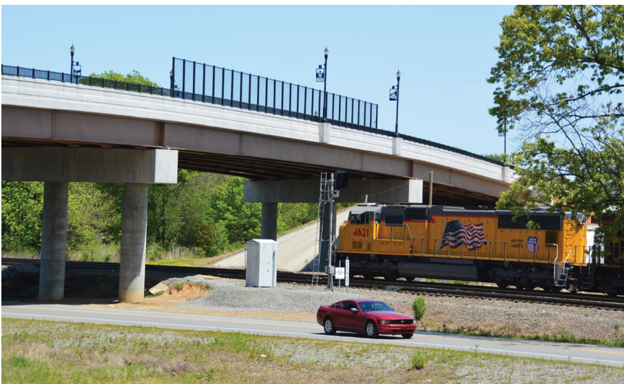
Rail grade separations, like the one on McCain Blvd., allowed major roads to safely span busy railroads, easing traffic flow and enhancing safety.
